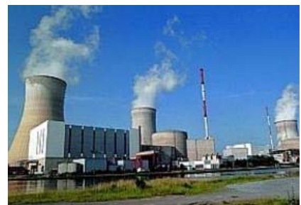
Tihange NPP site – general view
