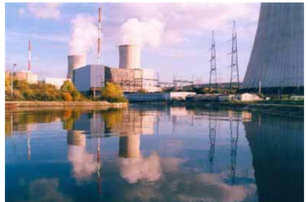
Tihange NPP site – general view
